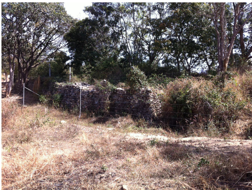
Electric fence backed by stone wall in Bannerghatta National Park, Karnataka, India. Photo by Heidi S. Riddle
